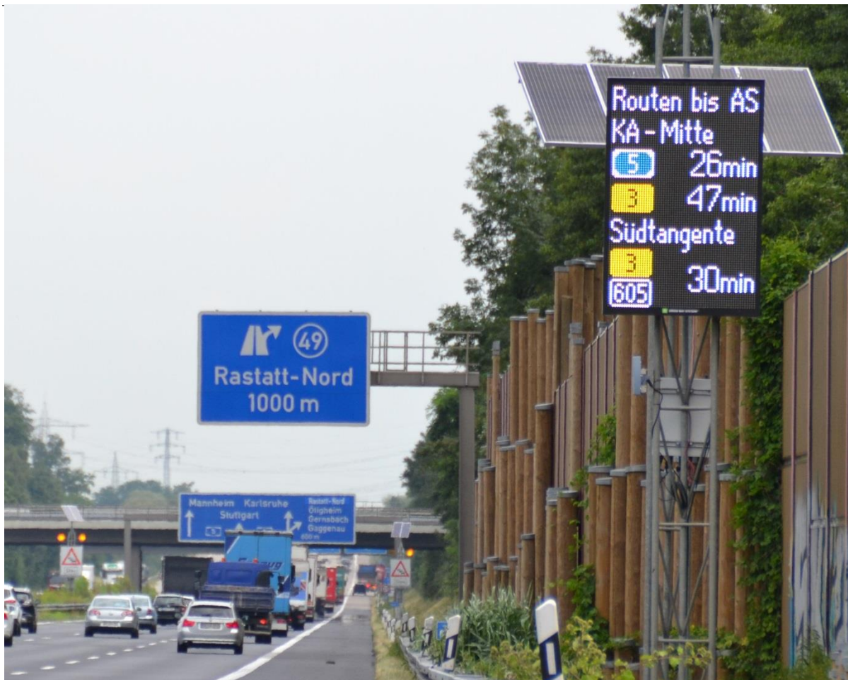
Picture 2: alternative routes are displayed ahead of the construction site (Source: Green Way Systems)
